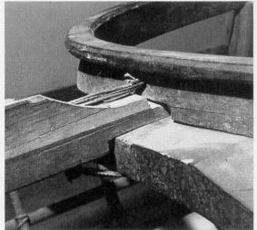
every 5 centimeters, just below it. Make sure none go through a saw kerf. Bring out the needle and waxed cord again, and sew or lash the lip in place. You can cut grooves across the top to countersink the lashings, but since this area will later be covered by canvas, it's not really necessary.
