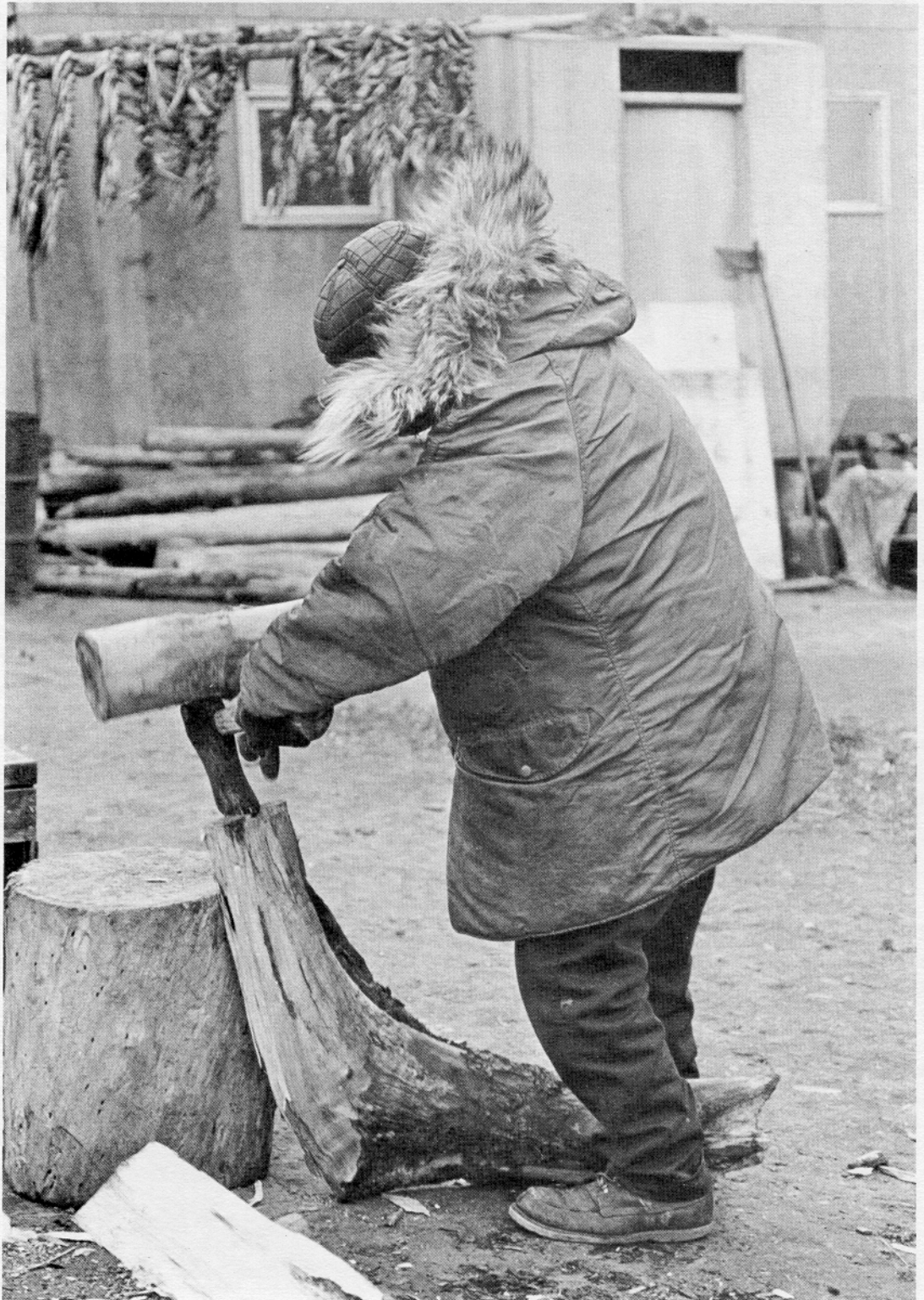
Figure 5. Dick Bunyan splitting a driftwood stump for kayak deck beams.
