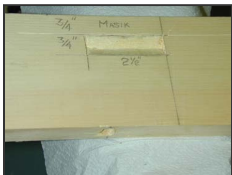
Figure 18. Deck beam finished mortise for masik .
