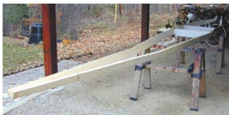
Figure 20. Gunwales spread apart with temporary masik and itivik - from bow.
