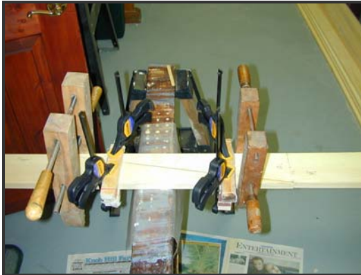
Figure 7. Setting up the gunwale scarf joint.
