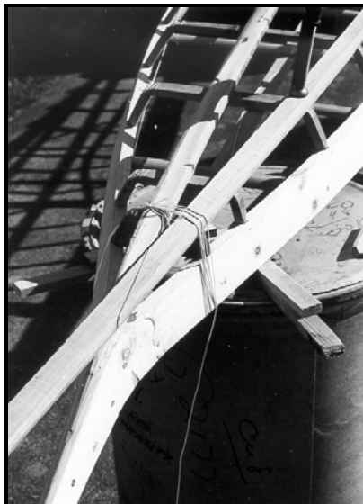
Figure 65. Aft bilge stringer being cut to fit.
