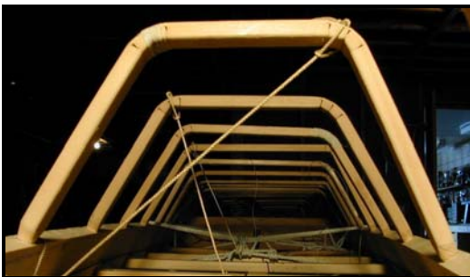
Figure 53. Rib in place with adjusting twine.
