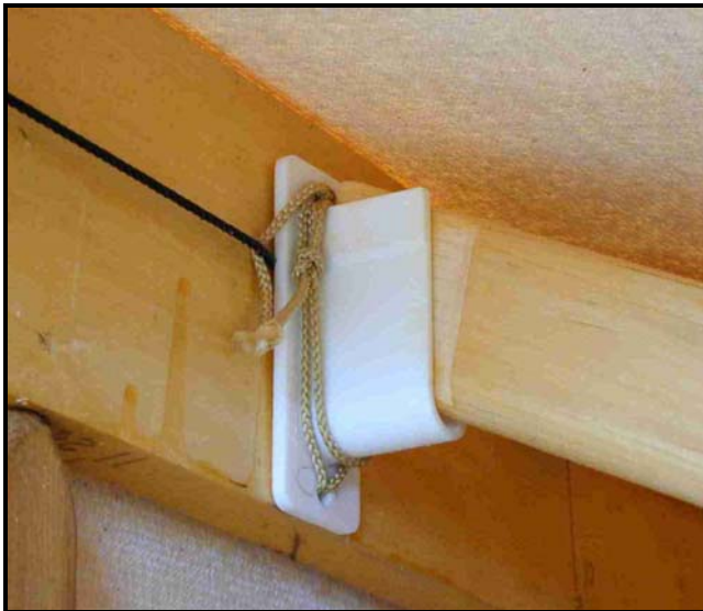
Figure 74. Foot brace installed.
